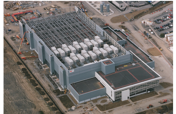
Microsoft Data Center (Dublin, Ireland)
