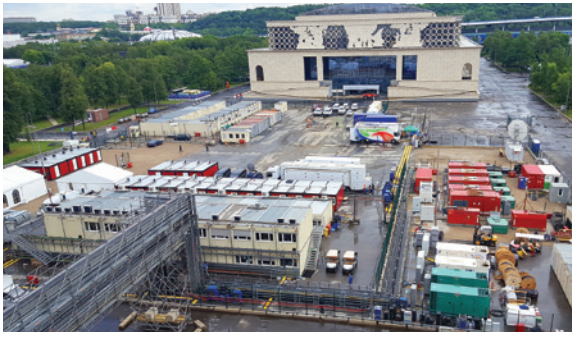
Luzhniki Main Stadium TV Compound 전경
